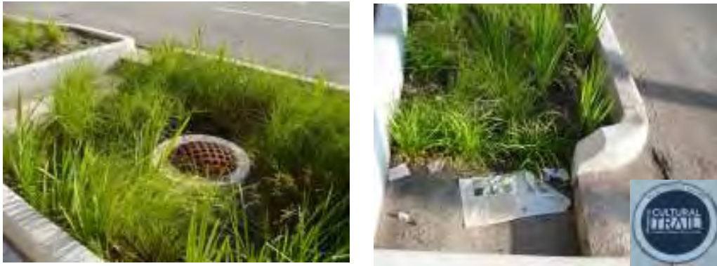
Curb Inlet, Pre-treatment and Raised Outlet for Indianapolis Cultural Trail Bioretention (Alabama Street)
