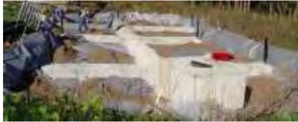
INSTALLATION OF BIORETENTION UNDERDRAIN
