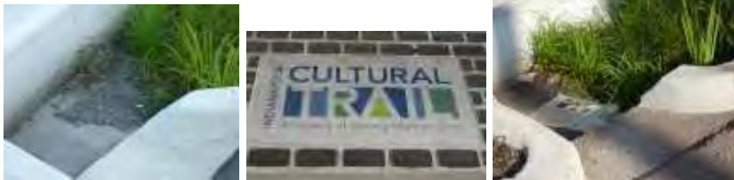
PRE-TREATMENT IN INDIANAPOLIS CULTURAL TRAIL BIORETENTION (ALABAMA STREET)
