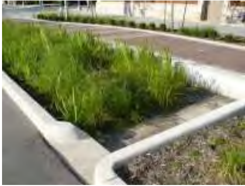
CURB CUT INLET – INDIANAPOLIS CULTURAL TRAIL BIORETENTION (ALABAMA STREET)
