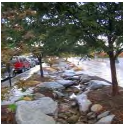
ALTERNATIVE “STREAM BED” URBAN BIORETENTION
